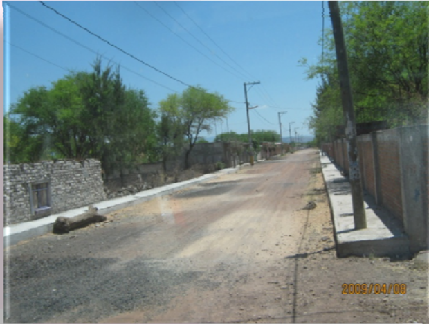
Electricity at León Cárdenas, Álvaro Obregón County, Michoacán / Club León Cárdenas (HTA), Chicago
